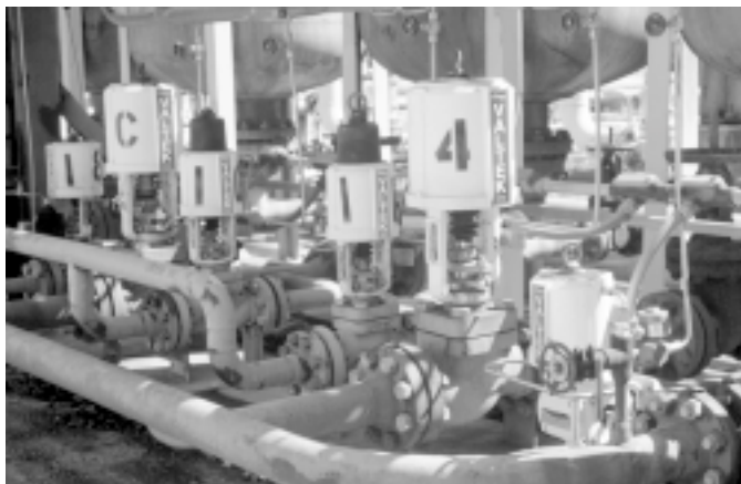
This cryogenic Mark One is used for aerospace testing as an O 2 vent valve.
